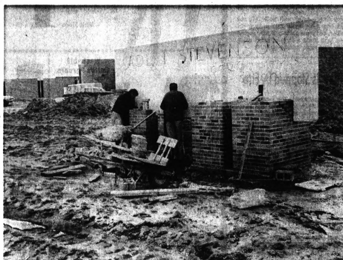
FINAL TOUCHES—Workers add the last bricks and mortar to the cement slab marking Adlai Stevenson High School in Utica. The school, which has an enrollment of about 1,300, opened today.
