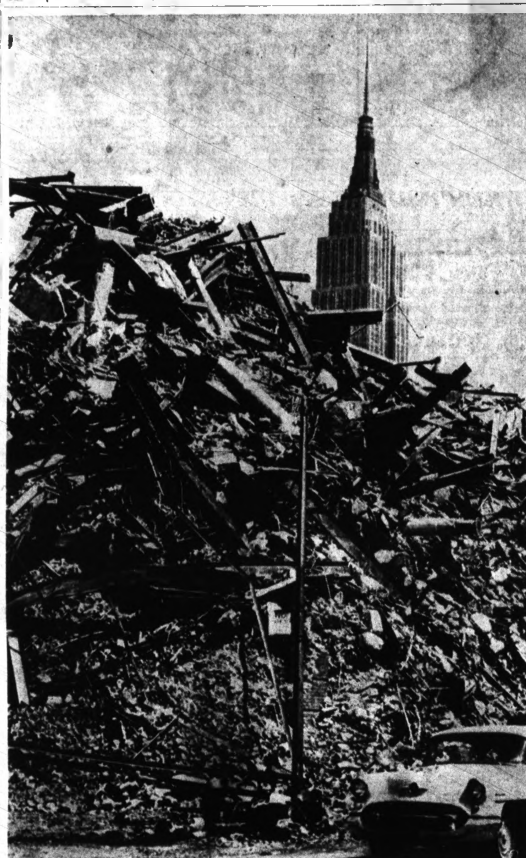
A HEAP OF LIVING—All New York appears to be in ruins as this towering pile of rubble seems to bury the Empire State Building, far in the background. The mountain of bricks and girders and wood is all that remains of hundreds of buildings demolished in a six-square-block area between Eighth and Ninth avenues, and
