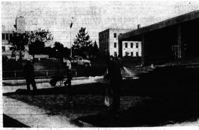
SODDING LIBRARY LAWN —Parks & Recreation Department workers laying sod and watering it in advance of the opening of the new Pontiac Public Library building later this month.
