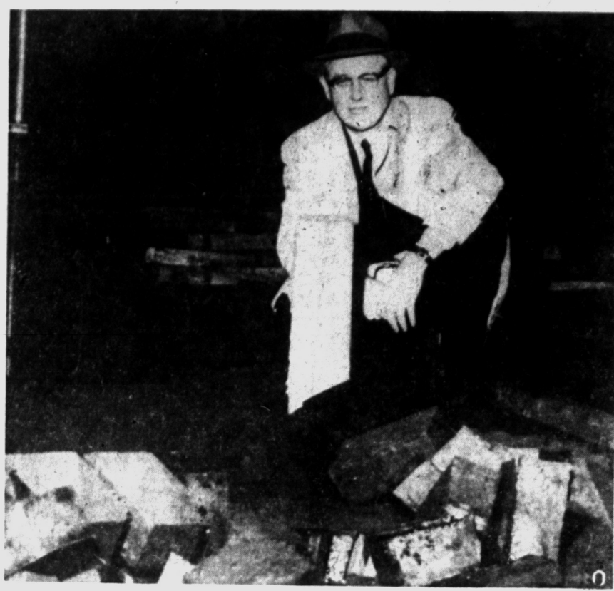
IDLENESS IS THE SINNER — Great Lakes Steel Corp. President W. D. MacDonnell inspects brick floor damage that has been caused by the steel strike, now in its 110th day. Moisture and falling temperatures on the building and equipment have caused open hearth furnaces to tumble in, floors to buckle and equipment to rust.
