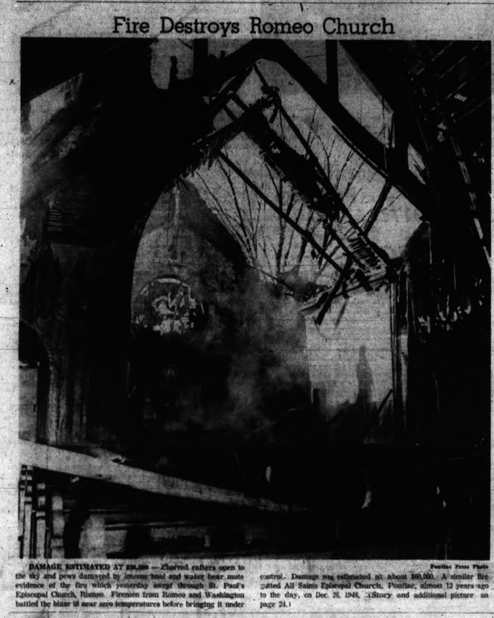
DAMAGE ESTIMATED AT $2000—Chaired rafters open to the sky and pews damaged by intense heat and water bear mute evidence of the fire which yesterday swept through St. Paul's Episcopal Church, Romeo. Firemen from Romeo and Washington battled the blaze in near zero temperatures before bringing it under control. Damage was estimated at about $2000. A similar fire gutted All Saints Episcopal Church, Pontiac, almost 12 years ago to the day, on Dec. 28, 1948. (Story and additional picture on page 24.)
