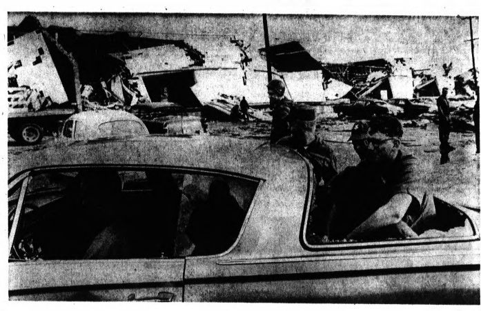
Passengers Get Open-Air View Of Gulfport, Miss., Wreckage
