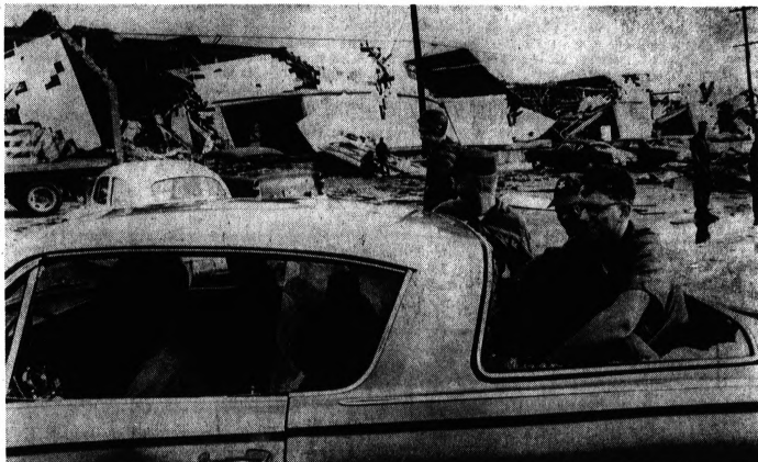
Passengers Get Open-Air View Of Gulfport, Miss., Wreckage
