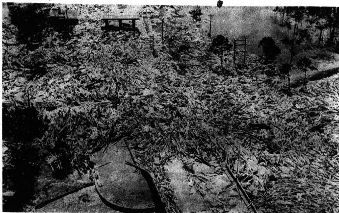
Debris Covers Bridge At Bay St. Louis, Miss.
