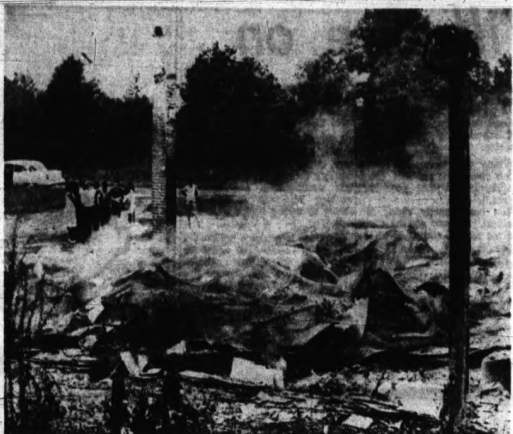
REMAINS OF CHURCH — The ruins of the Mount Mary Baptist Church smoldered amid racial unrest in Sasser, Ga., a town near Albany. The fire Sunday was blamed on segregationists. Another Negro church a few miles away was damaged by flames. At nearby Dawson, Ga., gunfire tore into a house Thursday and wounded a young white man, a member of an interracial group working to register Negro voters.
