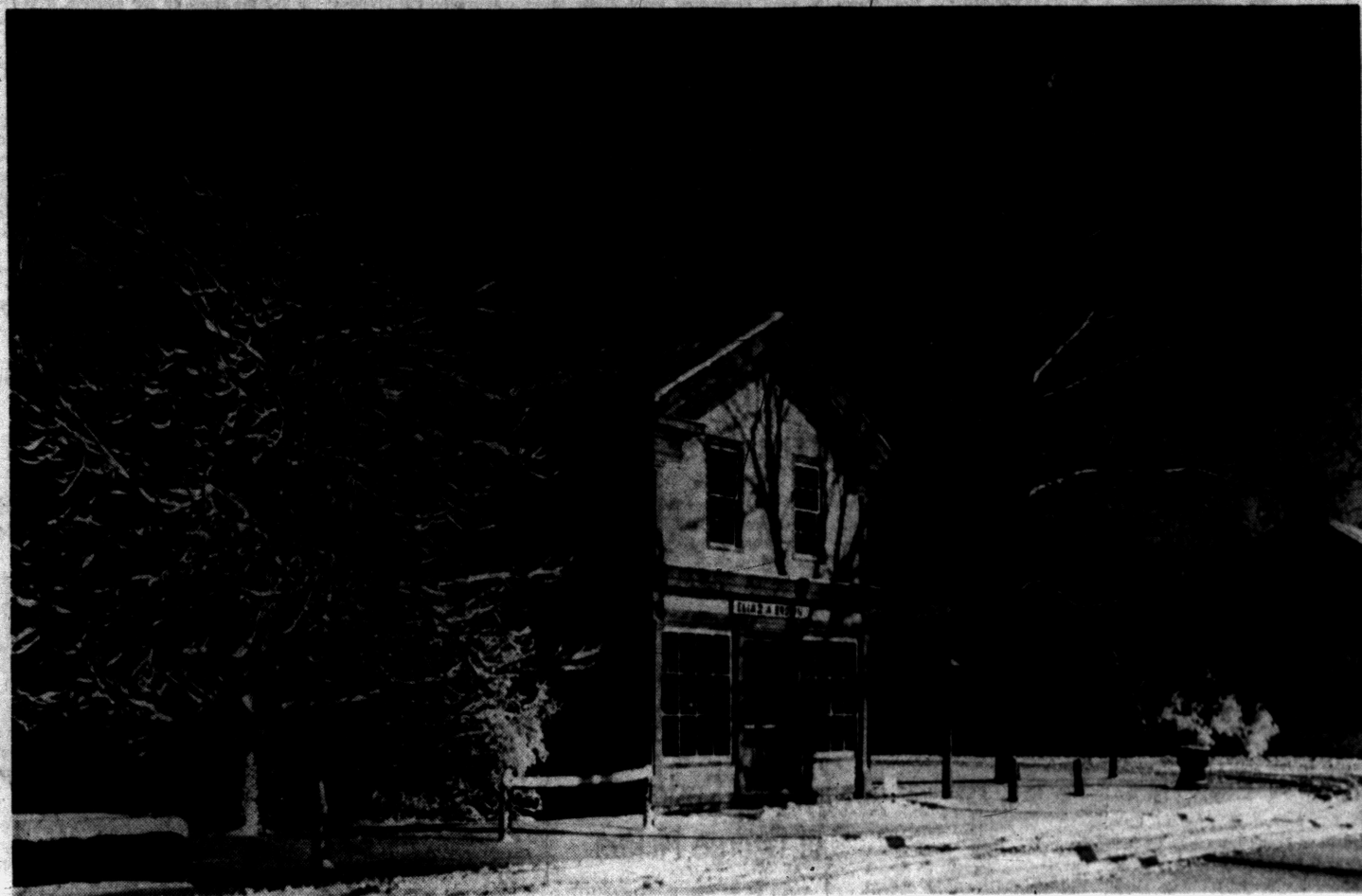
TRANSPLANTED — Snow, applied by the brush of Artist Winter, gives a picturesque appearance to the Waterford General Store, now located on the green at Greenfield Village in Dearborn. Built in Waterford in 1854, the old-time business establishment was a place where everything from drugs to dry goods and household
