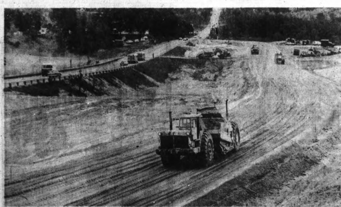
GROUNDWORK FOR FREEWAY — Preliminary work for the $11.5-million Pontiac-to-Orion M-59 freeway is well under way, as shown by this view of M-34 (Opdyke) south of Featherstone. Machinery in the foreground is building up the roadbed for temporary relocation of Opdyke. The short detour will carry traffic around construction of an overpass which will carry Opdyke over the new freeway.
