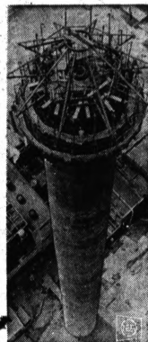
MISSILE MIGHT? — No, it's only a more than 400-foot-high smokestack at a Chillicothe, Ohio paper mill. The stack, tallest in the U.S. paper industry, was built at a rate of about 20 feet a day.
