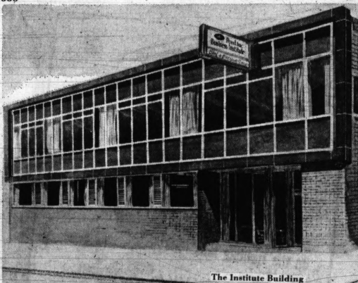
The Institute Building
