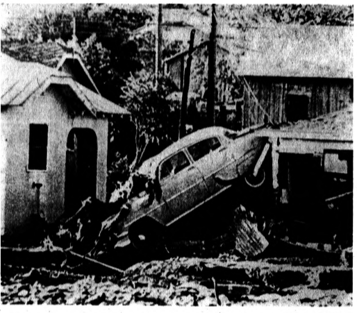
FLOOD DAMAGE — Floodwaters, sweeping through the west Texas town of Sanderson yesterday, pushed homes together, destroyed vehicles and buildings, and scattered debris for miles down normally dry Sanderson Canyon.
