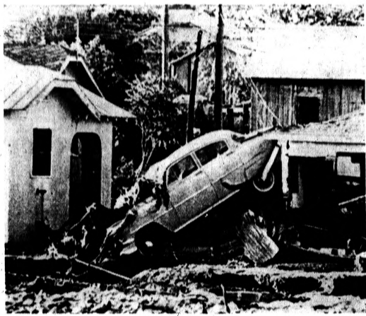
FLOOD DAMAGE — Floodwaters, sweeping through the west Texas town of Sanderson yesterday, pushed homes together, destroyed
