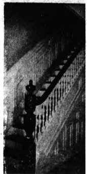
OLD STAIRCASE turns out to be a beauty when refurbished.
