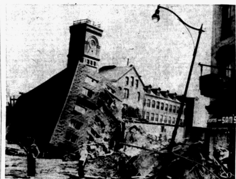
CHANGE OF ADDRESS—An apartment house once located on River Street in Waterbury, Conn., and housing 16 families lies crushed and broken at the intersection of River and Bank Streets, a block from its former site after flood waters of the rampaging Naugatuck River receded. Tower in background is that of American Brass Co. plant.
