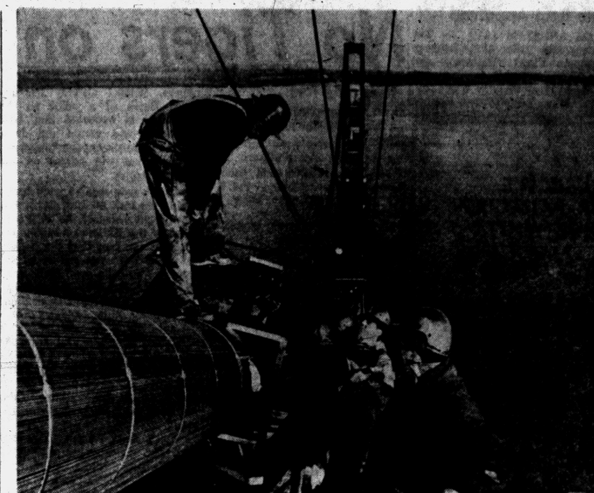
DANGEROUS PHOTOGRAPHY—Cameramen worked on swaying catwalks high above the Mackinac Straits to film "The Five Mile Dream," story of the world's longest suspension bridge, now showing at the Strand Theater, along with "This Happy Feeling," starring Debbie Reynolds.
