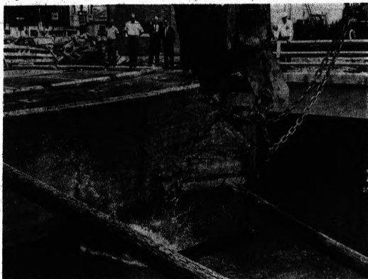
KERPLUNK — For several years, large wooden beams have kept this wall along the Clinton River just south of East Pike from "collapsing." Engineers predicted the wall, which leans toward the river, would come tumbling down when the beams were removed.
