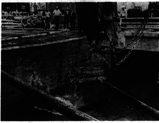
KERPLUNK — For several years, large wooden beams have kept this wall along the Clinton River just south of East Pike from "collapsing." Engineers predicted the wall, which leans toward the river, would come tumbling down when the beams were removed Friday afternoon by contractors improving the Clinton River. Here, the first of several beams is snapped by a crane. The engineers gathered to watch, and went away slightly baffled. The wall still stands.
