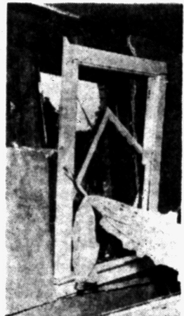
NEXT DOOR—Force of the blast tore out window frames in the apartment building adjacent to 6-8 Liberty St. Picture above was taken in the apartment building.
