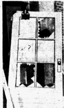
FRONT DOOR MOVED—This door to the adjacent apartment building was torn from its frame and left leaning by the entrance, as shown above, when the blast demolished the two-story house next door.
