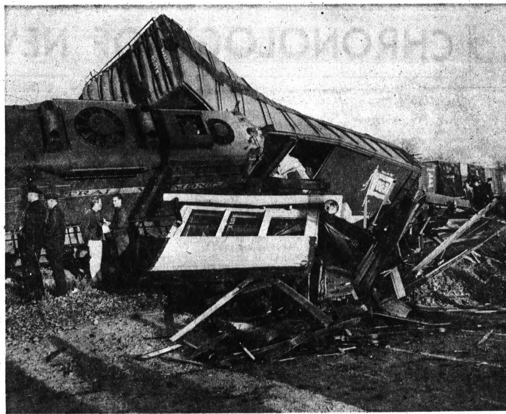
TRAIN WRECK — An observation tower was leveled and a switchyard employee suffered a broken leg when two diesel engines collided and one of them tipped over near a city crossing Oct. 29. The crossing area on North Johnson was
