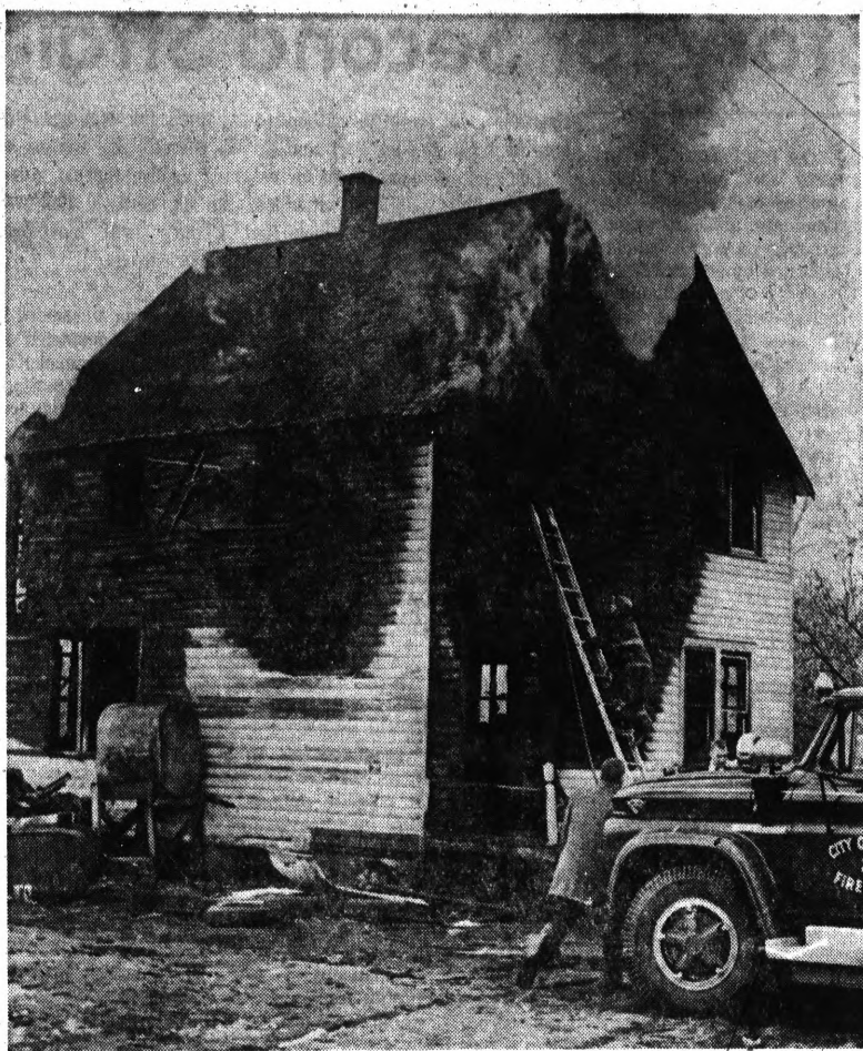
WHERE FOUR DIED — With smoke still billowing from an upstairs window, Troy firemen inspect the home of Mr. and Mrs. David Kirby of 6729 John R, after fire gutted the
