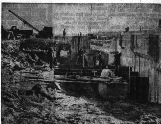
DETROIT WATER COMING —Construction of the Detroit Water Board service building in Troy is well on its way toward completion today. Located at the southwest corner of South Boulevard and Dequindre Road, the facility will be used to pump Detroit water to Pontiac and other northern Oakland County communities. The structure must be half-completed by November, according to stipulations of the federal grant with which it is being partially financed.
