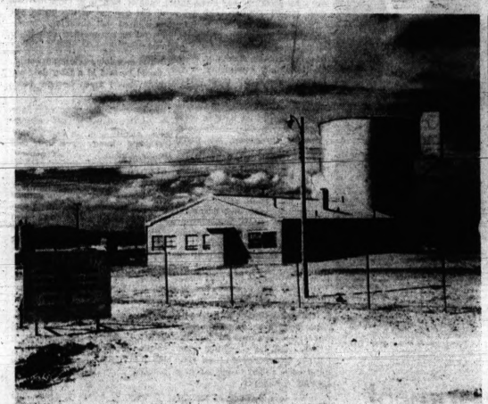
SITE OF EXPLOSION — In the basement of this building 40 miles from Idaho Falls, Idaho, a prototype of a small nuclear power plant blew up Tuesday night killing three military trainees, the only one in the building at the time. The blast was confined to the basement, and the area immediately surrounding it was filled with dangerous radiation. The Atomic Energy Commission has sealed off the area and says that neither the rest of the station or the town of Idaho Falls is in danger. The reactor involved is a forerunner of one planned for use by the Army in remote areas.
