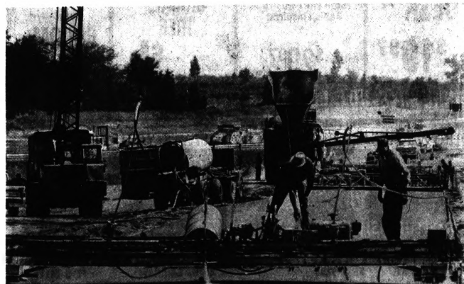
Chemicals Are Sprayed On Surface Of Wet Concrete To Make It Set Faster
