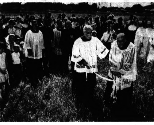
GROUND-BREAKING CEREMONY —Rev. Arthur Oldani (left), pastor of St. Vincent de Paul Catholic Church, helps Rev. Richard Thomas, pastor of St. Benedict's Catholic Church, dig the first shovelful of dirt at the new school site.
