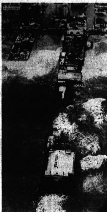
STEEL PIER DAMAGED —Seas rage around Atlantic City's famed Steel Pier after winds and waves gouged out a section of the resort attraction during the storm that has been spreading destruction along the Atlantic Coast for the past three days. The Boardwalk can be seen at the top in front of resort hotels surrounded by water.
