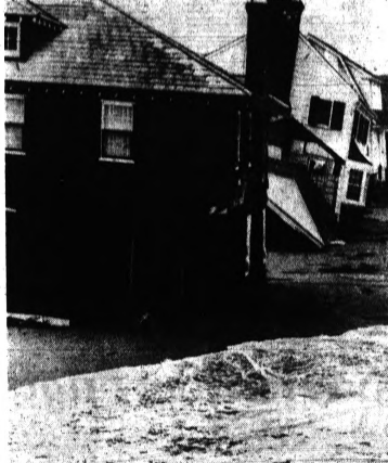
WEATHER WRECKAGE —Oceanfront homes at Virginia Beach, Va., tilt severely after extensive battering by high tides pushed ashore by gale winds Wednesday. City officials declared a state of emergency and called in the National Guard to prevent looting. The Red Cross, police and civil defense workers were operating in many of the stricken areas.
