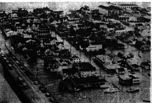
COAST CITY AWASH —Aptly named Ocean City, Md., is almost completely flooded Wednesday, forcing 1,000 residents to evacuate. The Sinepuxent Bay Bridge at the left now
