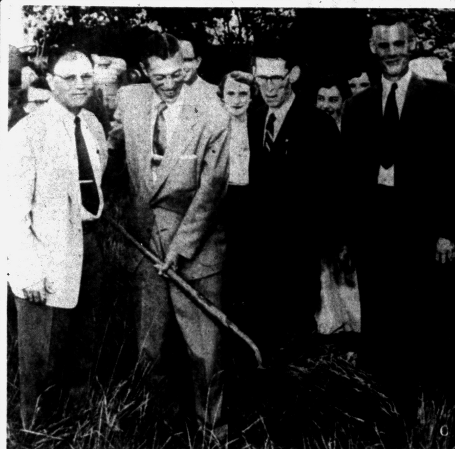
FIRST SHOVELFUL — Turning the ground at a ceremony held Tuesday night to initiate the site preparation for Rochester's new million dollar high school is Leonard J. Harding, president of the board of education. Shown also in the above photo are, left
