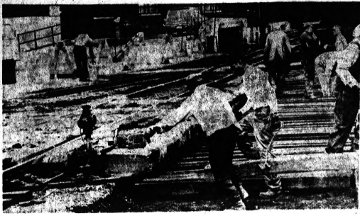
ALL THE LIVE-LONG DAY — As the familiar song goes, that's how crews are working on the Grand Trunk Western Railroad crossing on Oakland Avenue just south of Sanderson Street. Workmen are shown here placing new ties in the
