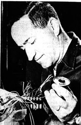
WIRE TROUBLE — Dawsey Forbis of 4134 Baybrook, Waterford Township, unscrambles wiring in the electrical shop of the maintenance department. Full-time employees repair record players and movie projectors as well as perform other electrical chores throughout the system.
