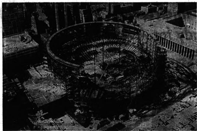
GARDEN GROWS — This bowl of steel built over the tracks of the Pennsylvania Railroad and the wreckage of the Old Penn Station outlines the shape of New York's new Madison Square Garden. The new Garden, to be used for
