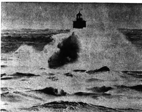
LIGHTHOUSE UNDER ATTACK — High seas thrown across a breakwater by blustery winds almost hide the Racine, Wis., North
