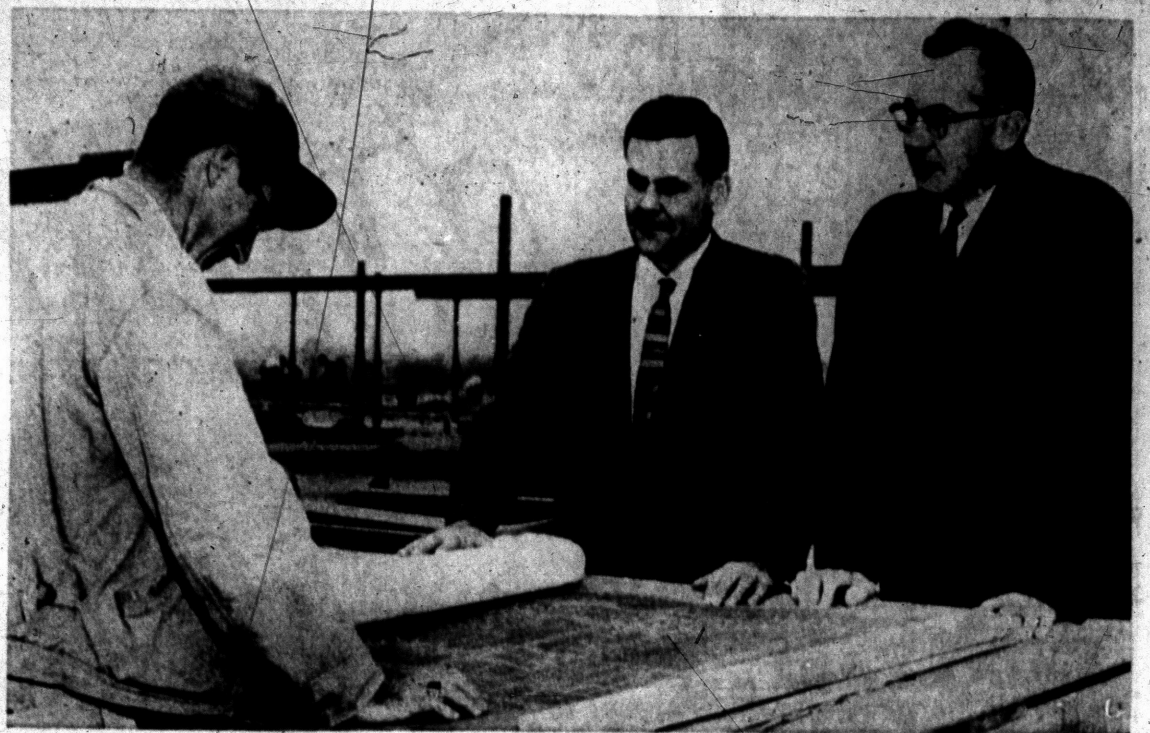
CHECK PROGRESS —Jim Loviska, carpenter foreman, looks over the plans of Pontiac's new high school with Dr. Dana F. Whitmer, (center) superintendent of schools and Glenn H. Griffin, president of the board of education. The school, now under construction (in background) on Arlene street between Madison and Perry streets, is expected to be ready by September 1958. Cost of the building is more than $3 million. It will have an initial capacity of 800 students.
