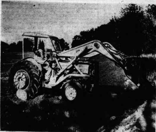
PARK PROJECT STARTED — Clearing land at the site of the Stony Creek Metropolitan Park development northeast of Rochester is George Hock of 4650 Inwood Road, Washington Township.
