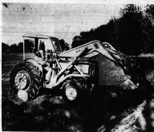
PARK PROJECT STARTED — Clearing land at the site of the Stony Creek Metropolitan Park development northeast of Rochester is George Hock of 4050 Inwood Road, Washington Township.
