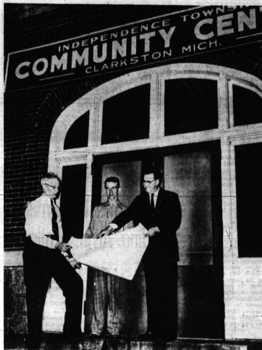
CENTER REFURNISHED — Independence Township officials look over plans for renovation being completed on the 50-year-old community center in Clarkston. All of the floors in the 2-story structure have been refinished, revealing golden-burled maple under layers of varnish. New cupboards have been installed and painted in the kitchen. Other rooms also have been repainted and new lighting fixtures installed. Pictured (from left) are Kenneth Johnson, township treasurer; Harold Doebler, clerk for 25 years; and Supervisor Duane Hursfall. Cost of the project is about $2,000.
