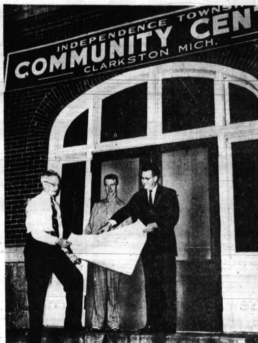
CENTER REFURBISHED — Independence Township officials look over plans for renovation being completed on the 30-year-old community center in Clarkston. All of the floors in the 3-story structure have been refinished, revealing golden hued maple under layers of varnish. New cupboards have been installed and painted in the kitchen. Other rooms also have been repainted and new lighting fixtures installed. Pictured (from left) are Kenneth Johnson, township treasurer; Harold Boeber, clerk for 25 years; and Supervisor Duane Hurstall. Cost of the project is about $2,000.
