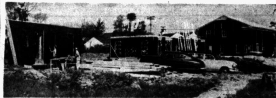
MORE HOUSES —As the expansion from the metropolitan area continues to spill into Oakland County, these new homes are under construction in Bloomfield Township. Building permits total $3,860,000 so far this year. The total reached $9,810,600 in 1953.
