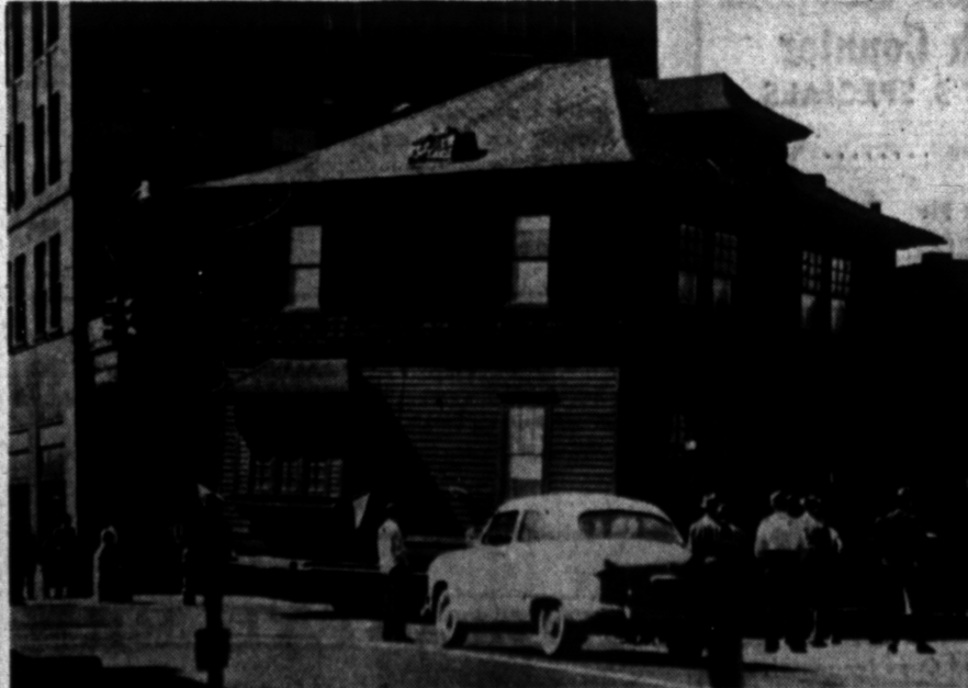
MOVING DAY—The home of the late Judge Charles P. Webster is shown being moved today from 127 Wayne St., where it was erected about 40 years ago. It has been sold by Mrs. Webster to Warren LaLone, and goes to 2144 Garland Ave. in Sylvan Lake City, where it will be occupied by the LaLone family. Mr. and Mrs. Webster had occupied the house many years. Its former site will be used as a parking lot. The picture was taken just after the house entered West Huron street from Wayne.
