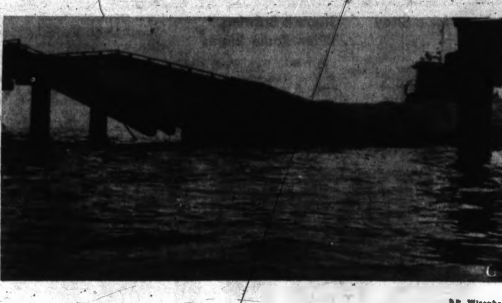
BRIDGE RAMMED — The Lake Pontchartrain Causeway, world's largest over-water bridge, was hit by a barge Wednesday in a black fog. Two 52-foot sections collapsed and bridge
