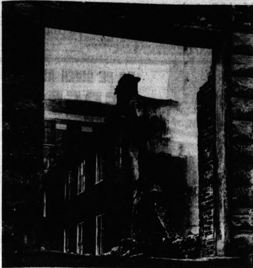
DOWNTOWN CLEARANCE —A picture window view of wrecking operations for Community National Bank's employee parking lot off Wayne Street in downtown Pontiac shows the exposed interiors of ancient buildings, dominated by the Riker Building garage (rear). The $75,000 clearance job is about half way done. About 100 parking spaces will be provided.
