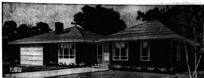
SOMETHING DIFFERENT: Similar pavilion roofs, with a small flat roof between, are combined with vertical redwood siding in this contemporary ranch to produce an eye-
