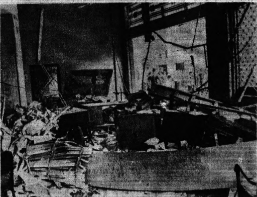
WRECKED INTERIOR — A crowd gathers outside the wrecked interior of the American Embassy's consulate section. A Viet Cong terrorist automobile blew up alongside the building with an estimated 250 pounds of explosives. The blast killed one terrorist. The other was shot and wounded by a Vietnamese policeman.
