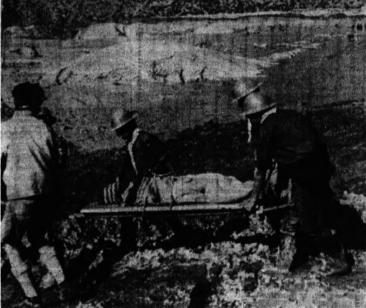
DISASTER AFTERMATH — Chilen Boy Scouts act as stretcher-bearers for one of the victims of yesterday's earthquake and flood. In the background is a sea of mud left when the quake split open a 230-foot-high dam to send millions of tons of water over the El Cobre, Chile, area. Approximately 400 were killed. (See story, Page 2).
