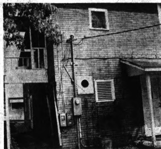
NEW LOOK — Exemplifying what can be accomplished through systematic code enforcement is this structure at 520 Franklin Road. The photo at left was taken last August.
