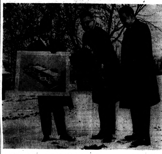
BREAK GROUND — Developer Harold Goldman (left), City Commissioner Robert C. Irwin and City Manager Joseph A. Warren broke ground yesterday for the first of four buildings in a 50-unit apartment complex on Wide Track near Cottage. Goldman expects his housing project to be completed by spring.
