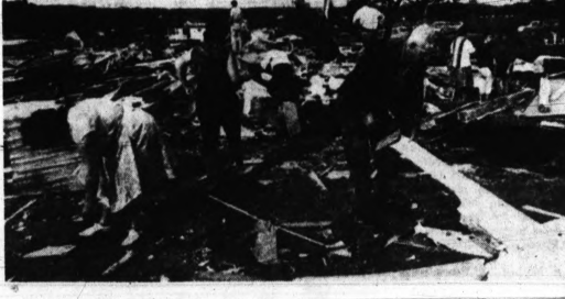
SCENES OF WRECKAGE — Seven houses were destroyed and several others damaged by a tornado which struck a housing development southeast of Rochester, Minn., yesterday. Thirteen persons were injured, none critically. In photo at top, a house has been moved off its foundation. Bottom picture shows residents picking up fragments of their demolished homes.
