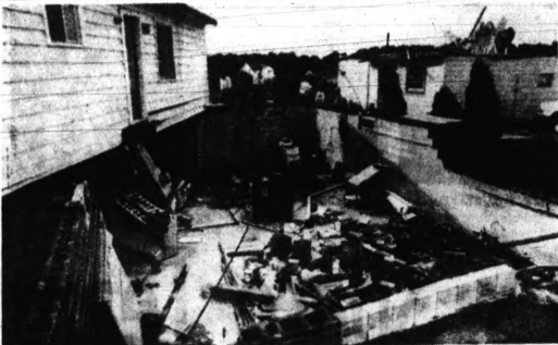
SCENES OF WRECKAGE — Seven houses were destroyed and several others damaged by a tornado which struck a housing development southeast of Rochester, Minn., yesterday. Thirteen persons were injured, none critically. In photo at top, a house has been moved off its foundation. Bottom picture shows residents picking up fragments of their demolished homes.
