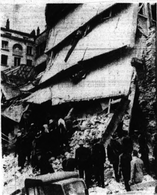
SEEK VICTIMS — Firemen and workmen search the wreckage of a government office building in Brussels, Belgium, that crumbled today, killing at least 10. Rescue operations were later halted because it was feared that the overhanging concrete slabs would fall on the diggers.
