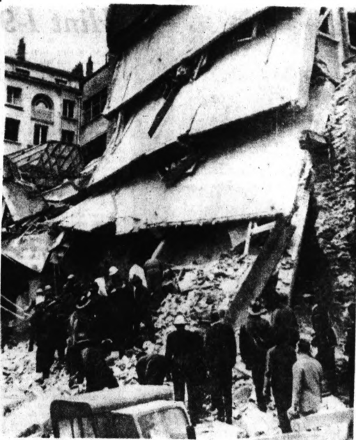
SEEK VICTIMS — Firemen and workmen search the wreckage of a government office building in Brussels, Belgium, that crumbled today, killing at least seven. Rescue operations
