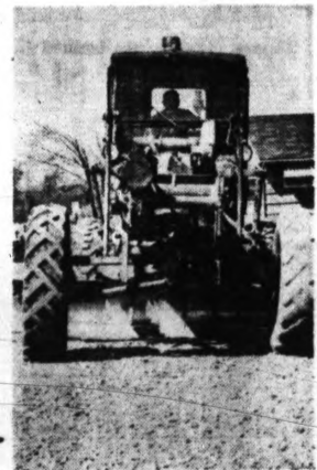
City forces graded, graveled and paved over 3 miles of city streets.
