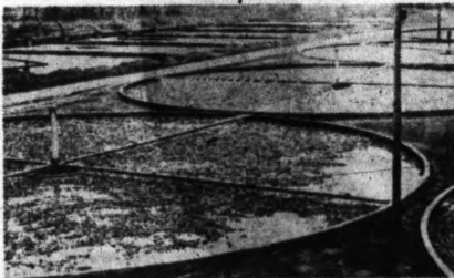
DEPARTMENT OF SEWAGE TREATMENT
