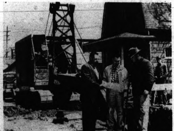
Step by step inspection of city construction insures safety and quality.
