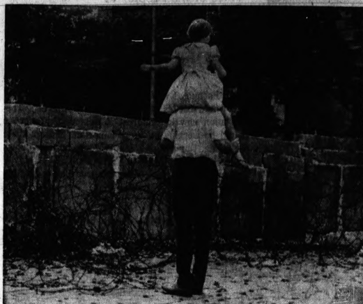
Cracks Appearing In Berlin Wall
