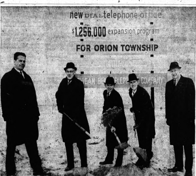
CONSTRUCTION STARTS — Breaking ground for the $1.25-million Bell Telephone Co. central office in Orion Township are (from left) E. Eugene Russell, the company's Pontiac district commercial manager; John Lessiter, Orion Township supervisor; State Rep. Robert J. Slingerland, D-Lake Orion; Earl J. Fortin, president of the Orion Area Chamber of Commerce; and Charles B. Woodhead, Michigan Bell Pontiac manager. (See story, Page A-4)
