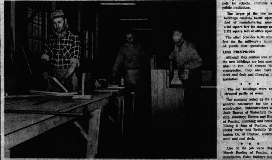
BACK AT WORK — Cabinetmakers are busy again at the Pontiac Millwork Co., only five months after the firm's facilities were totally destroyed by a spectacular fire. The millwork's back in full operation at two new buildings after a rapid recovery from the $500,000 blaze. The company specializes in custom doors and cabinets for schools, churches and public institutions.
