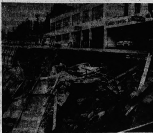
CAVE-IN CLOSES STREET —A cave-in tore up 90 feet of Fifth Avenue in downtown Seattle Wednesday and forced the closing of the thoroughfare between James and Cherry streets. A salesman, Frank J. Watson, 50, was in an auto
