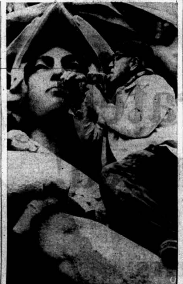
WHO CARES? — Looking off into the distance with complete indifference, this Parisian stone lady appears unruffled by the fellow working on her face with hammer and chisel. The figure, a fixture on Paris' Alexander III Bridge, is being readied for a forthcoming visit from the British Royal Family.
