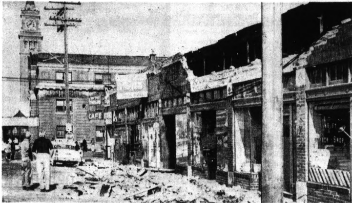
SEATTLE SHAKES UP — A street in downtown Seattle, Wash., is littered with bricks shaken loose by an earthquake today. This street is near the railroad station. Similar damage was reported over a wide area of the city.
