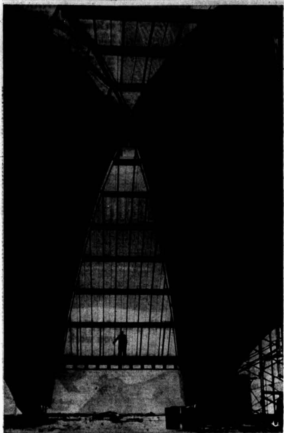
CATHEDRAL OF THE AIRWAYS —Lots of the "wild blue yonder" can be glimpsed through the new administration building at Lambert-St. Louis Airport, Mo. Workman, lower center, is installing aluminum frames for glass in the slat skylight. The $3,900,000 structure uses about 450 panes of specially cut glass ranging up to 68 by 123 inches in size. There are eight of the massive parabolic arches in the building.
