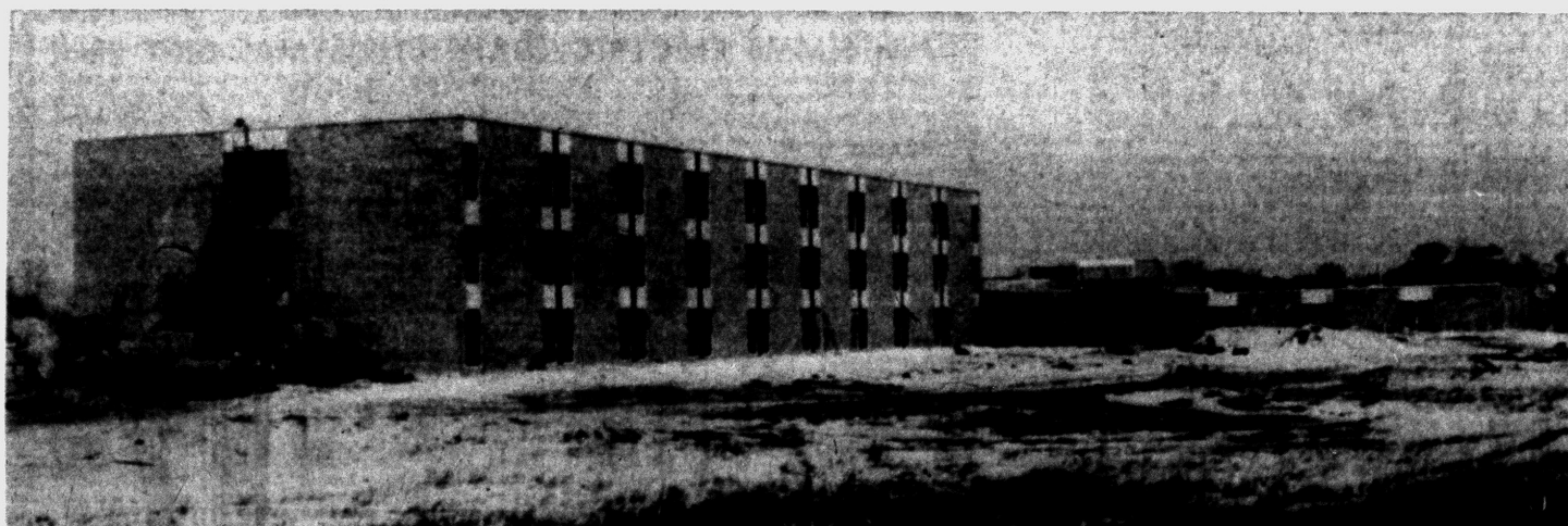
WALLS ARE UP—The first academic building on the campus of Michigan State University Oakland is right on schedule, according to George Karras, MSUO supervising engineer. Workmen are now installing windows in the building and putting up the interior walls. Roy Alexander, director of student affairs, said that facilities for closed circuit TV are being provided in all classrooms. MSUO is scheduled to open for a freshman class of 600 in September, 1959.
