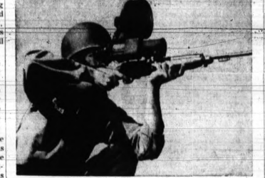
NEW SNIPERSCOPE —U.S. Army sharpshooter sights through a new infrared sniperscope which can spot a target far beyond the range of the World War II model. Developed by Raytheon, the new sight is scheduled shortly for large-scale production. Instead of the cumbersome World War II back pack, the entire power supply is carried in lightweight cartridge belt container.
