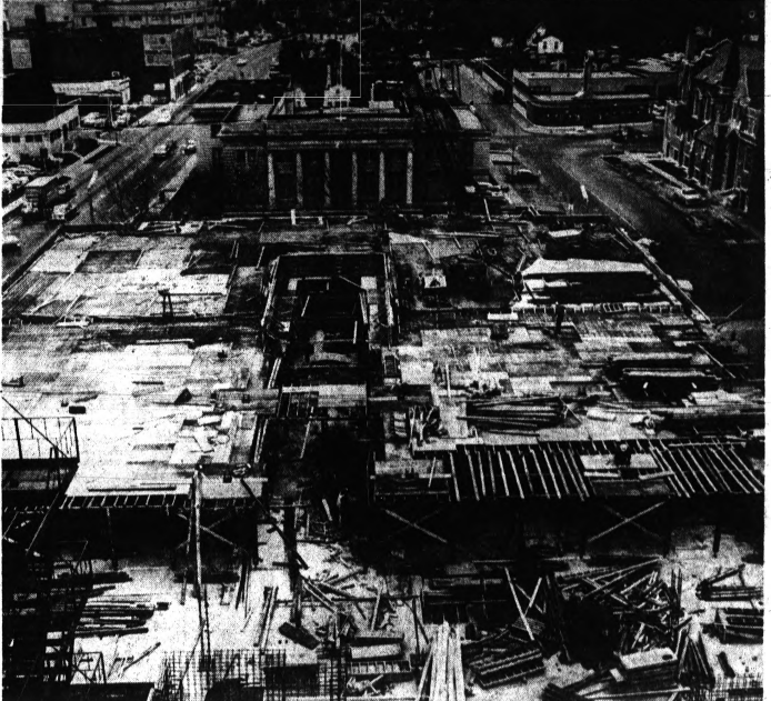
FROM THE TOP — Looking down from the top floor of the present Pontiac Osteopathic Hospital building, patients and staff members are confronted with this scene of activity. Workmen are
