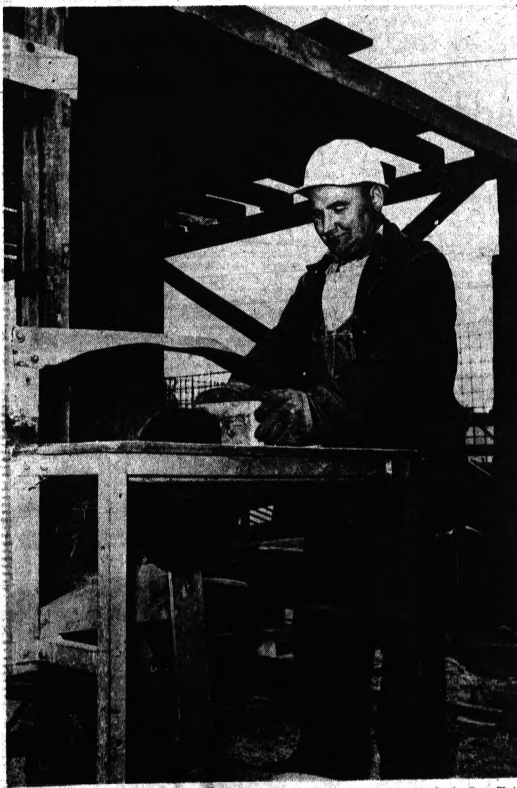
HE'S HELPING — Joe M. Rogers of 4510 W. Marcella St., Utica, is one of the construction workers working on the new osteopathic hospital addition. At present he and his fellow workers are ahead of their construction schedule.
