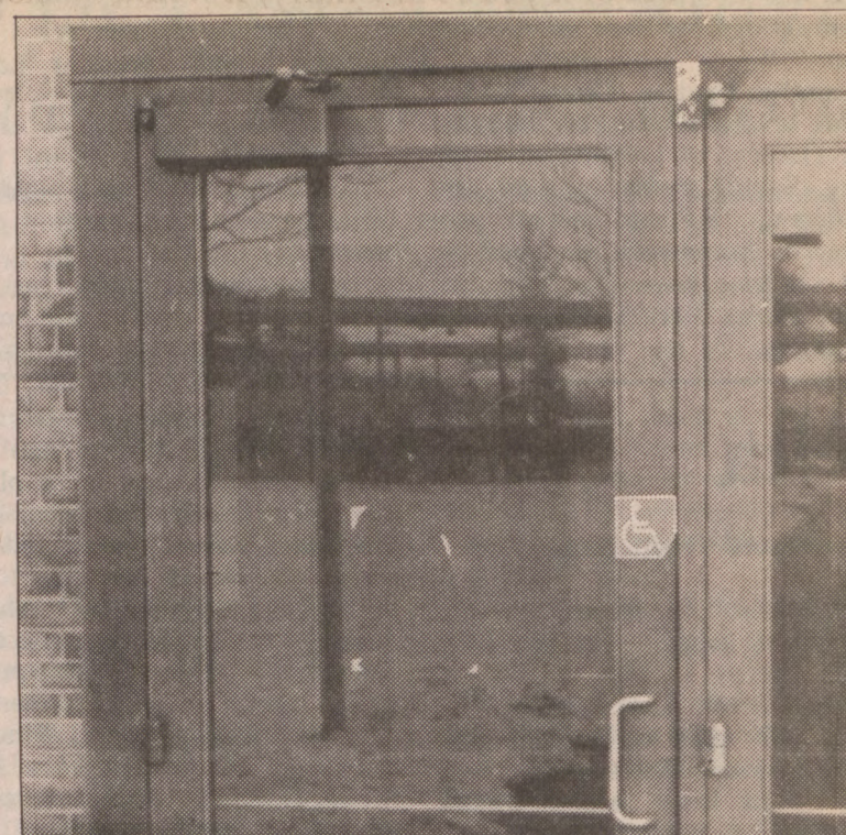
The Oakland Post/ Eric Kurtzy This automatic doors (this one is on the west entrance of the Oakland Center) work with remote control devices like garage door openers.
